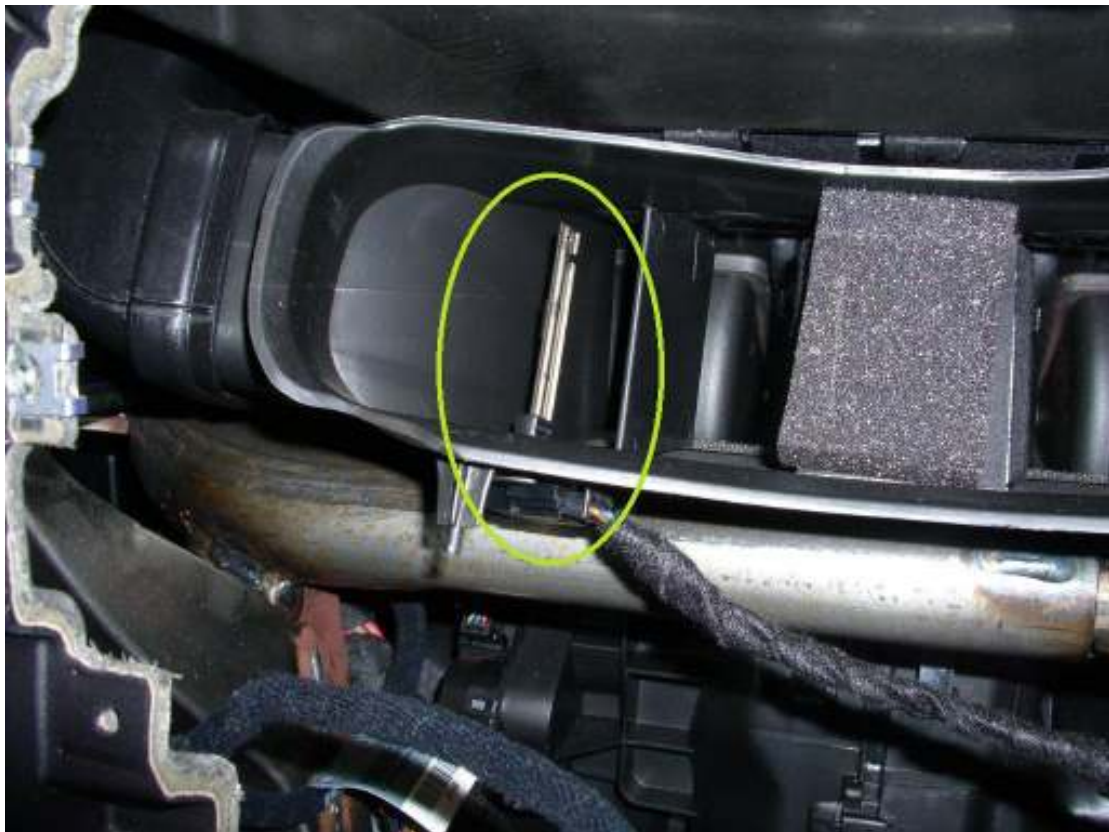
50. Central duct out. Disconnect 2 electrical connectors . Release 2 spring clips - press in to reduce the tension at the bottom then pop off the bottom with screwdriver.
